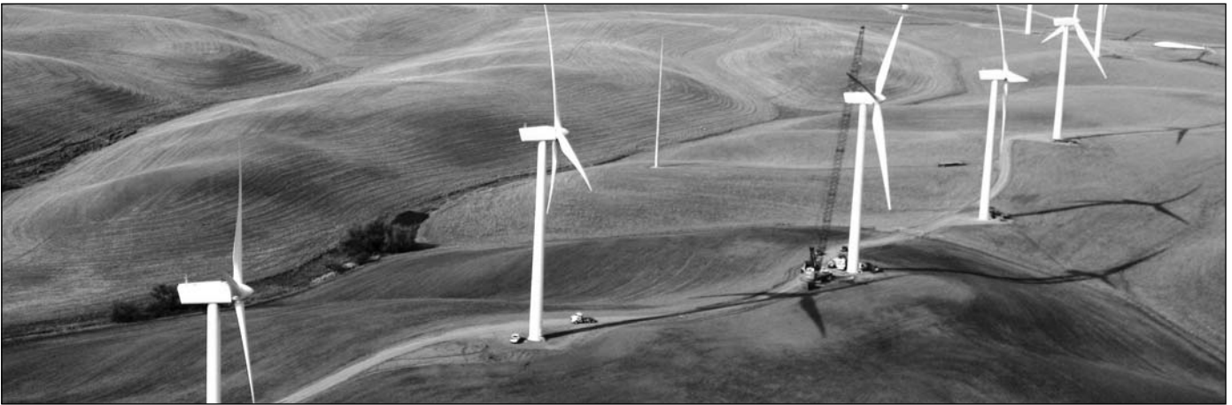
The Shiloh wind project in Solano County, Calif., will have an output of 150 MW when it is completed later this year. Photo courtesy of PPM Energy.
